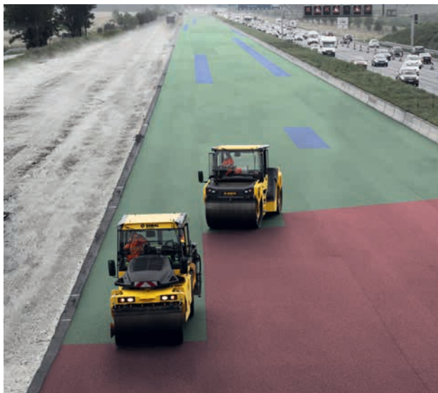
BOMAG technologies and assistance systems bring transparency to compaction results.
